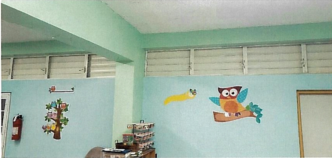
Photo #3 Short Column geometry. No damage was observed.
