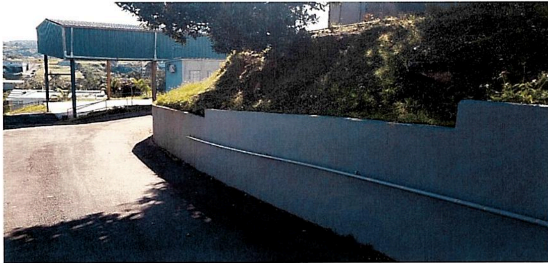
Photo #4 Retaining wall in good conditions.
