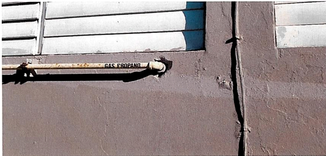
Photo #6 Jacketed Gas Entrance ok.
